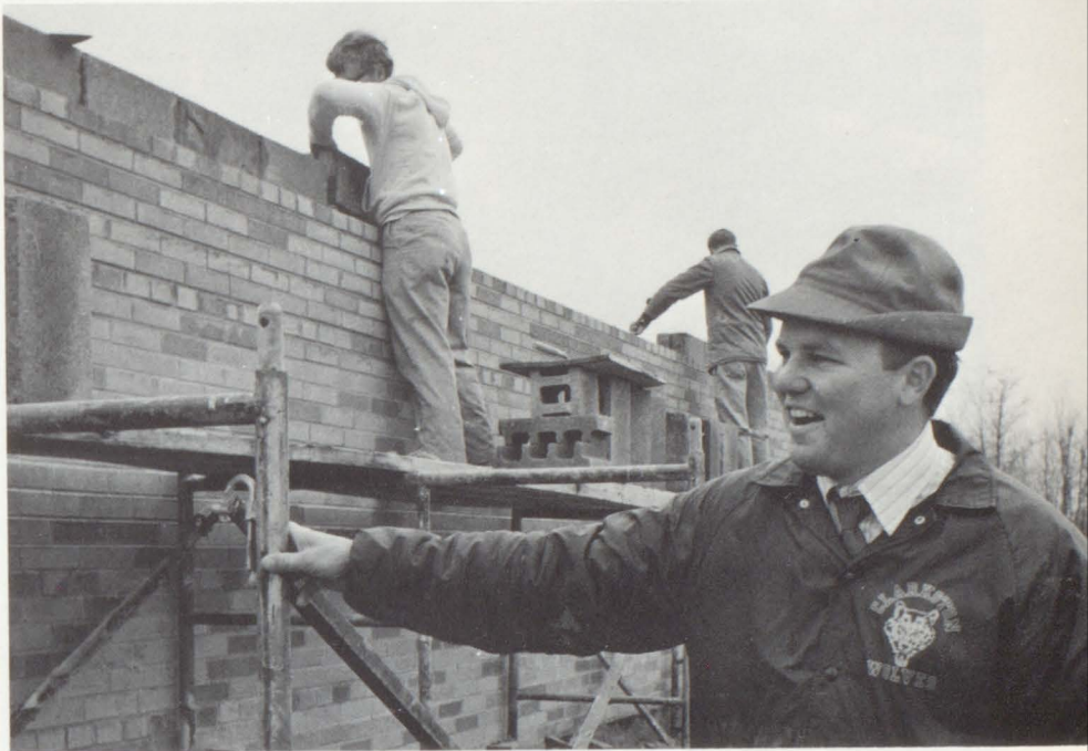
Mr. Bruce directs his construction class in building a new garage.
