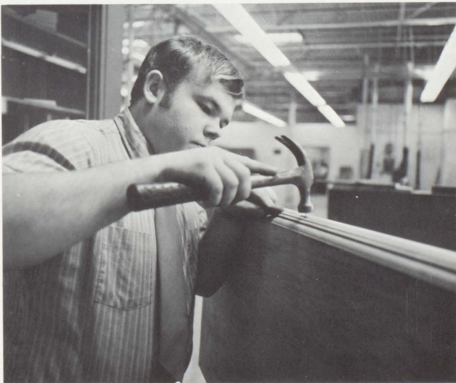
Mr. King puts the finishing touches on a building construction project.
