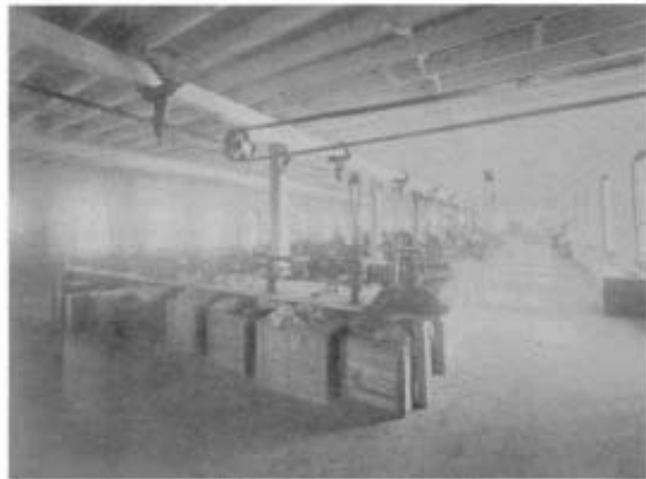
MACHINE ROOM WESTERN KNITTING MILLS.
