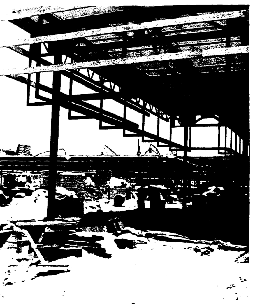
MIDDLE SCHOOL—Recent thefts and damage at Novi's middle school, under construction next to the high school, has resulted in a loss estimated at $2,500 (See story on Page 9-A). Work on the school reportedly is progressing satisfactorily despite the thefts, rain, and last weekend's blanket of snow.
