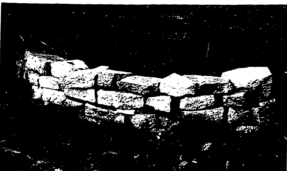
A WALL of un cemented stones or blocks does a good job of holding and concealing a compost pile. Structures should be located where they are easy to get to but not conspicuous. This one is located in an out-of-the-way corner along a backyard fence.
