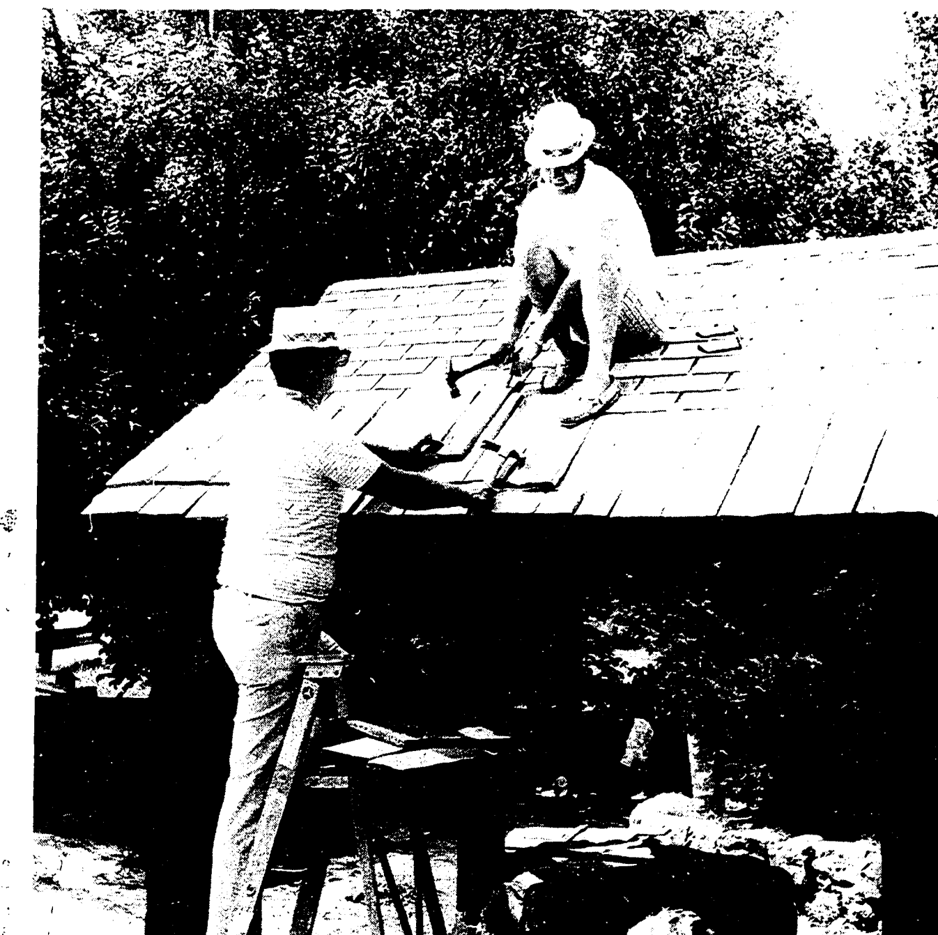
NEW ROOF —That's Northville Jaycee Don Campbell with the hammer putting a new roof on Northville's artesian well. Ron Beier is helping but prefers the step ladder. The result of their efforts last week was a new appearance to South Main Street's popular attraction.
