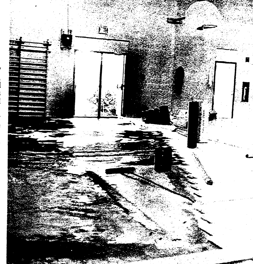
ON THE LEVEL—The gym floor at Cooke Junior High got a lift this week when emergency repairs were made to raise the sinking floor so the gym can be used when school opens. Similar measures were taken in the boys' locker room where the floor also has settled and walls cracked. Presently two Northville students is involved in a law suit against the architect, contractors and bonding company charging fill under the floor was not properly compacted. The floor has been sinking for the past two years.
