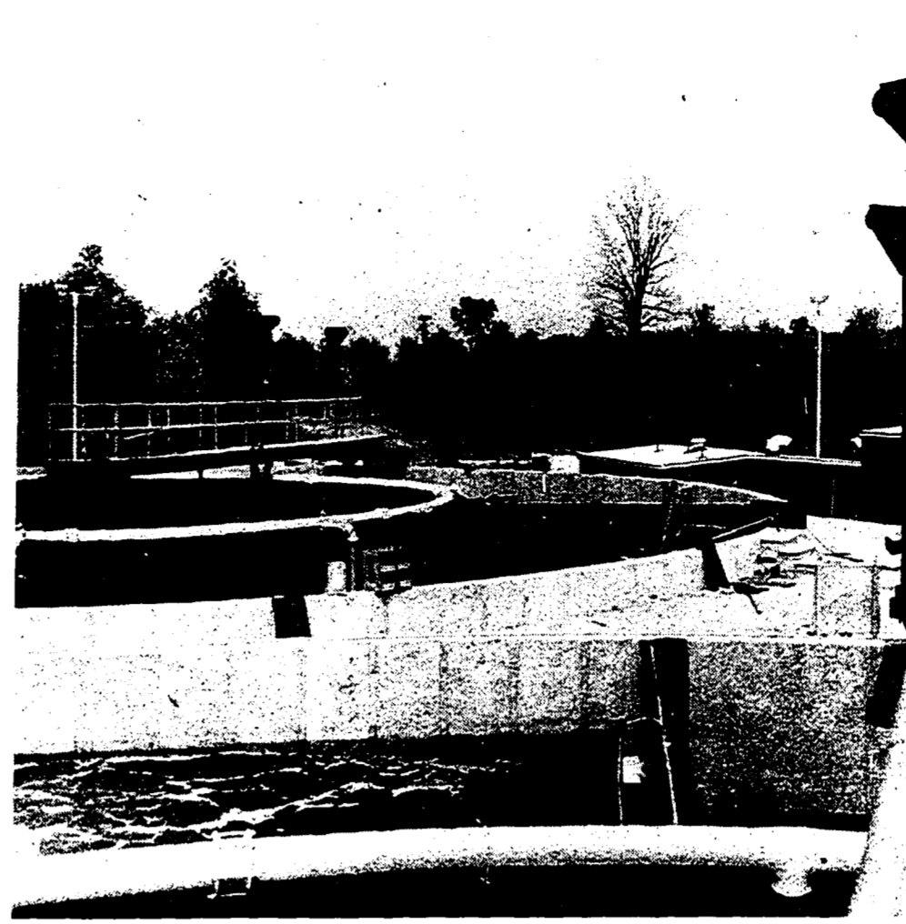
MILLION DOLLAR PLANT—The new Novi-Walled Lake sewage treatment plant is one of the most modern and efficient in the nation. Experts report that by the time the sewage has passed through the tertiary treatment system, it is 97 per cent free of impurities and is fit for drinking.
