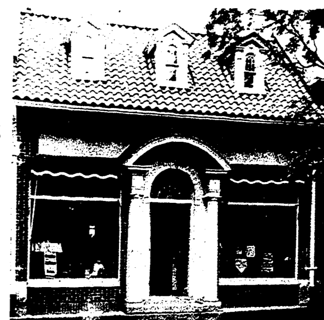
ORIGINAL OFFICE — Remodeled and now the quarters of Cloverdale Farms Dairy at 134 North Center Street, this building was the original Detroit Edison office about 1915. This picture shows how the building looked 50 years ago.
