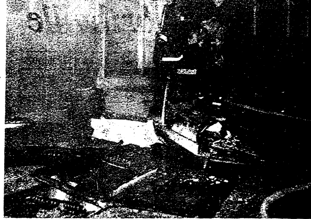
HOSPITAL BLAZE — Northville firemen remove rubble from Building D at Northville State Hospital after a fire early Tuesday gutted the storeroom and snack bar area. Heavy smoke and dense fog hampered firefighters who fought the 1 a.m. blaze. Patients were evacuated from the building but no injuries were reported. The fire is under investigation by the hospital's safety department and the State Fire Marshal's office.
