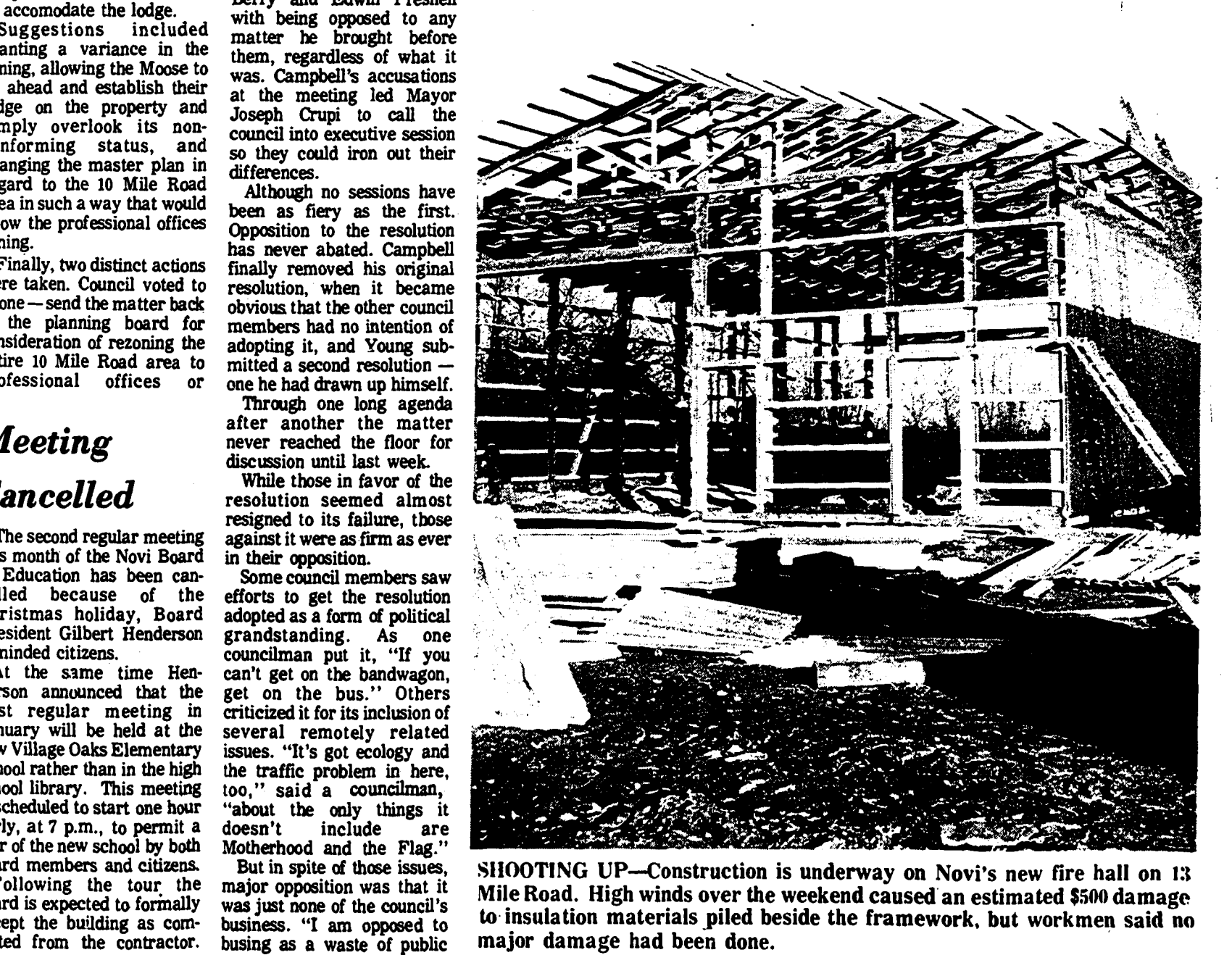
SHOOTING UP —Construction is underway on Novi's new fire hall on 13 Mile Road. High winds over the weekend caused an estimated $500 damage to insulation materials piled beside the framework, but workmen said no major damage had been done.
