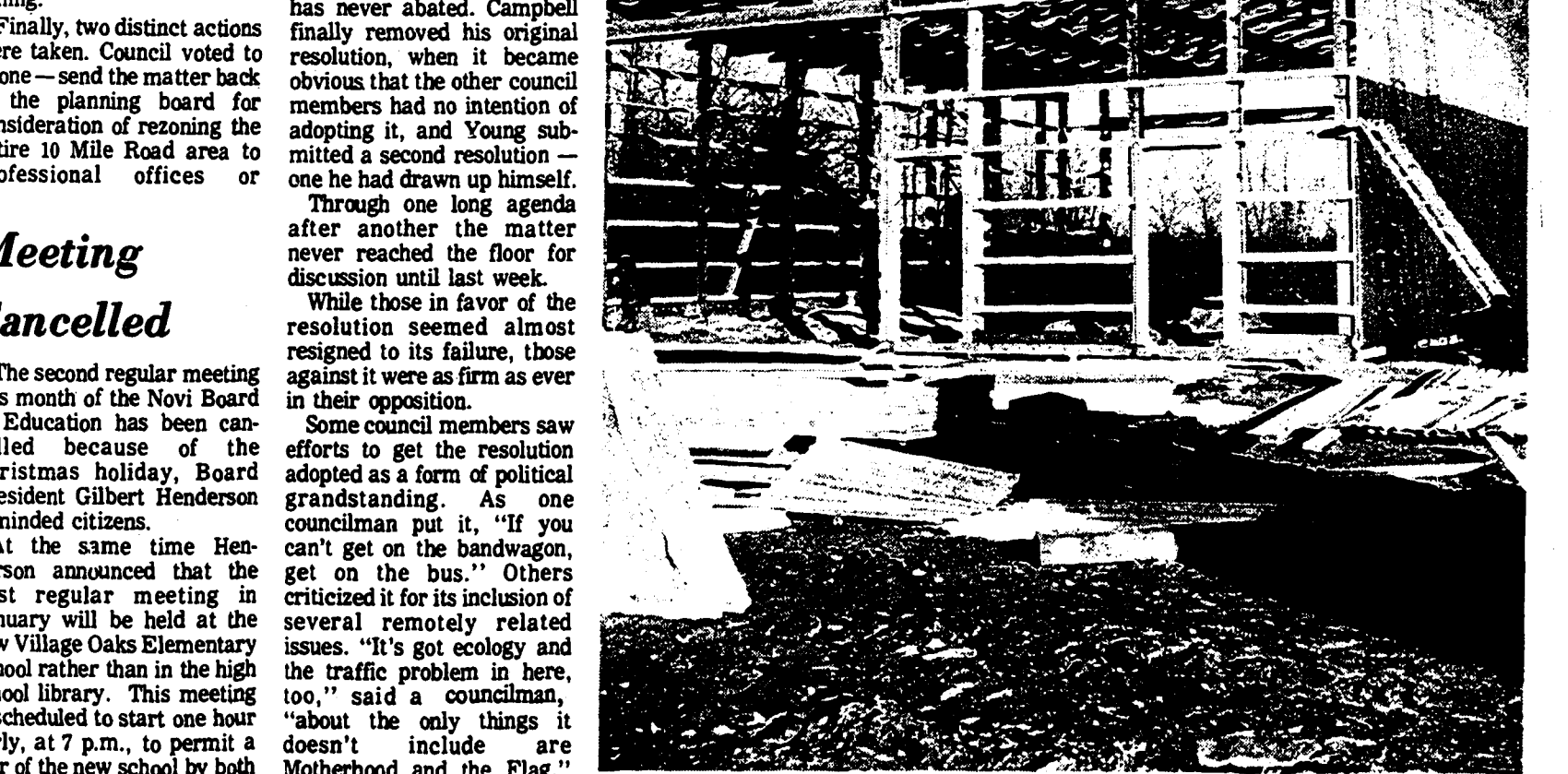
SHOOTING UP—Construction is underway on Novi's new fire hall on 13 Mile Road. High winds over the weekend caused an estimated $500 damage to insulation materials piled beside the framework, but workmen said no major damage had been done.
