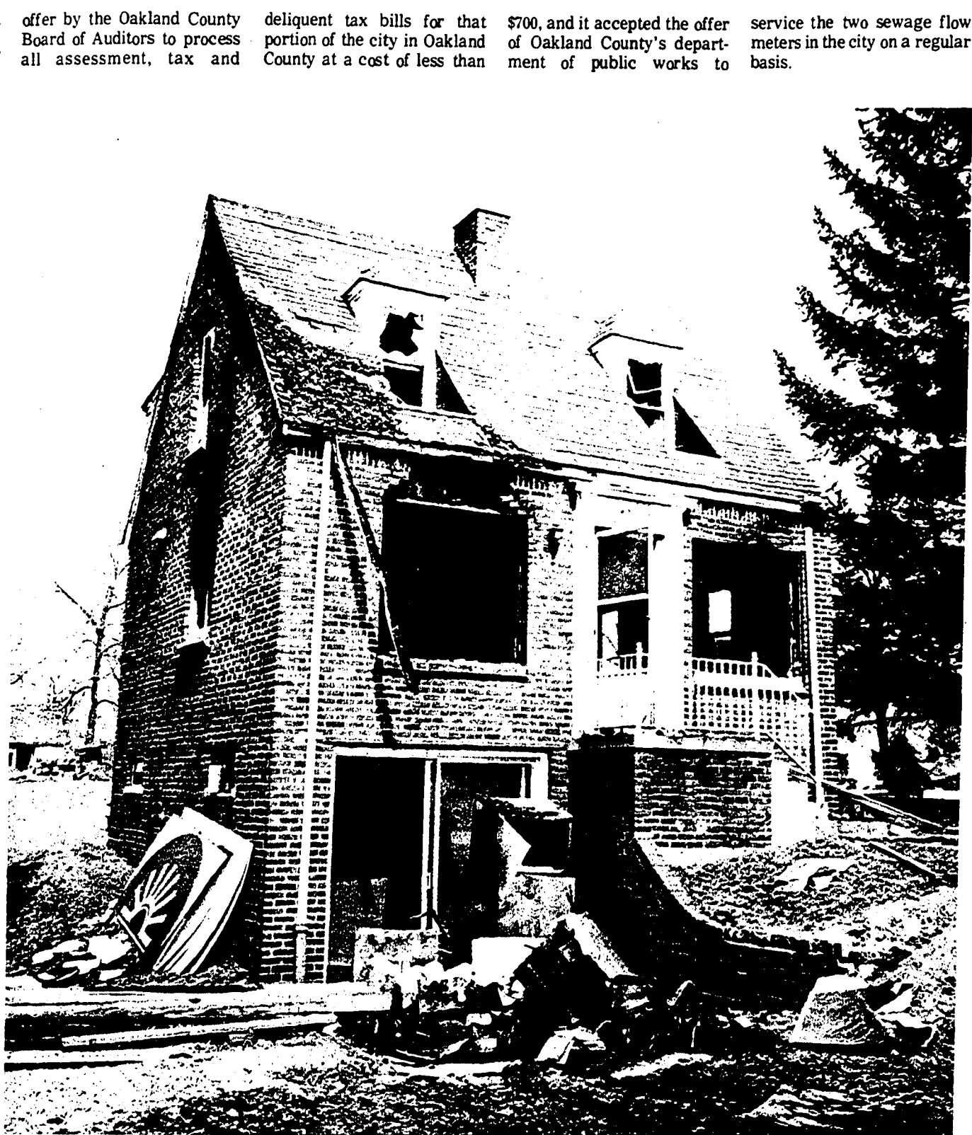
GUTTED —Levitt and Sons' construction office at 43000 Seven Mile Road was gutted by fire early Monday morning. Police have charged an escapee from Northville State Hospital with arson.
