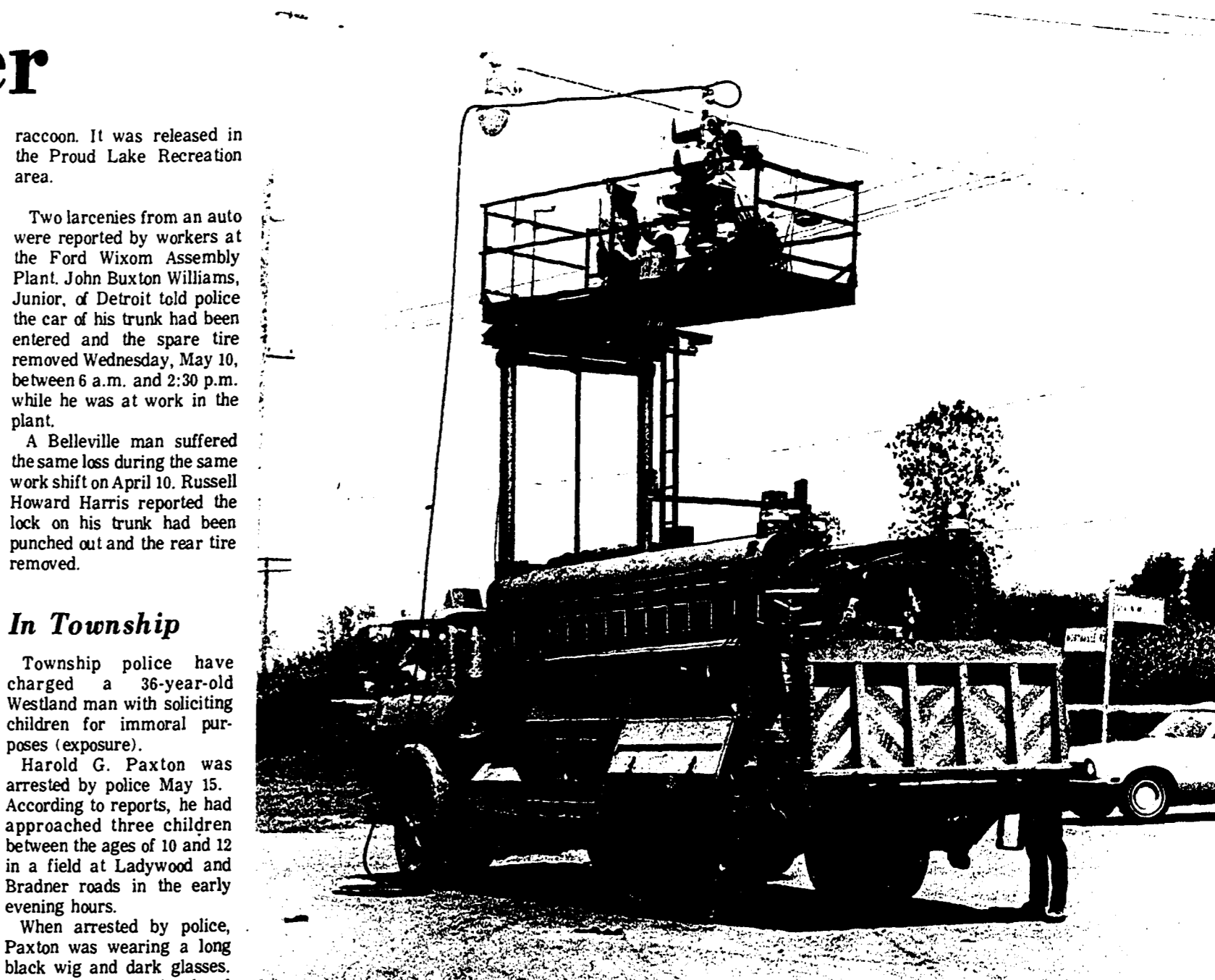
SIGNAL INSTALLED—After more than a two-year wait, a traffic signal was installed at Seven Mile and Northville roads Friday. The signal, temporarily only blinking a yellow caution, will become a conventional green-red light once motorists are accustomed to its location. Spearheading the light's erection was a Northville Township citizen, V. E. Clement, 1541 Jamestown, who fired off numerous letters and telephone calls to the county road commissioner before receiving assurance from Commissioner Philip Neudick that a light would be installed.
