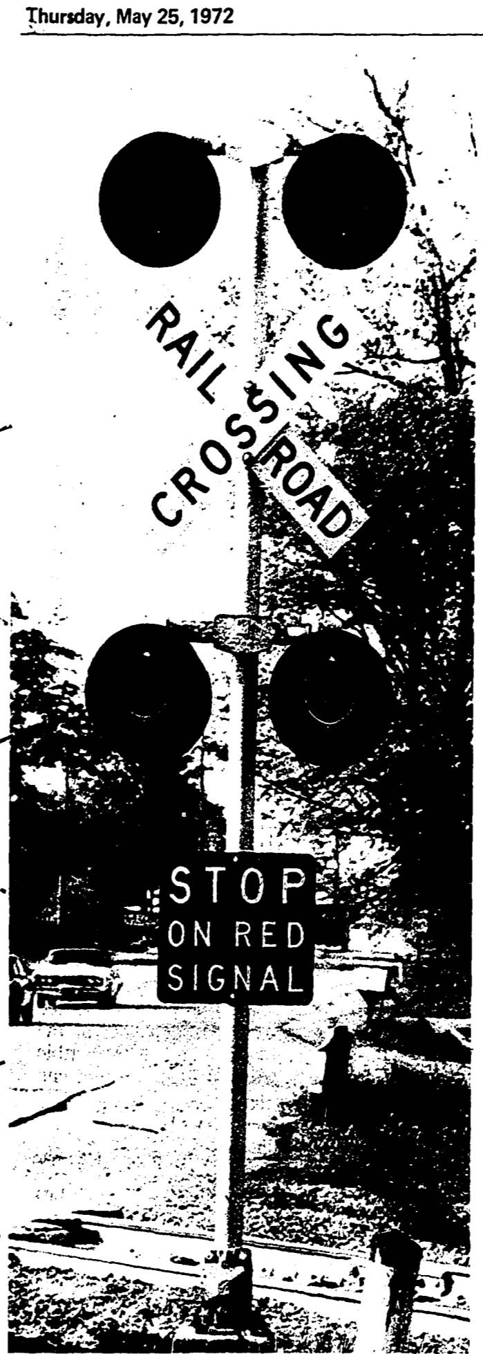
OVER THE HILL—New railroad flashers were installed on southbound Novi Road as a result of a Jaycee traffic safety project. The top set of flashers allows motorists to be warned well in advance of the crossing.
