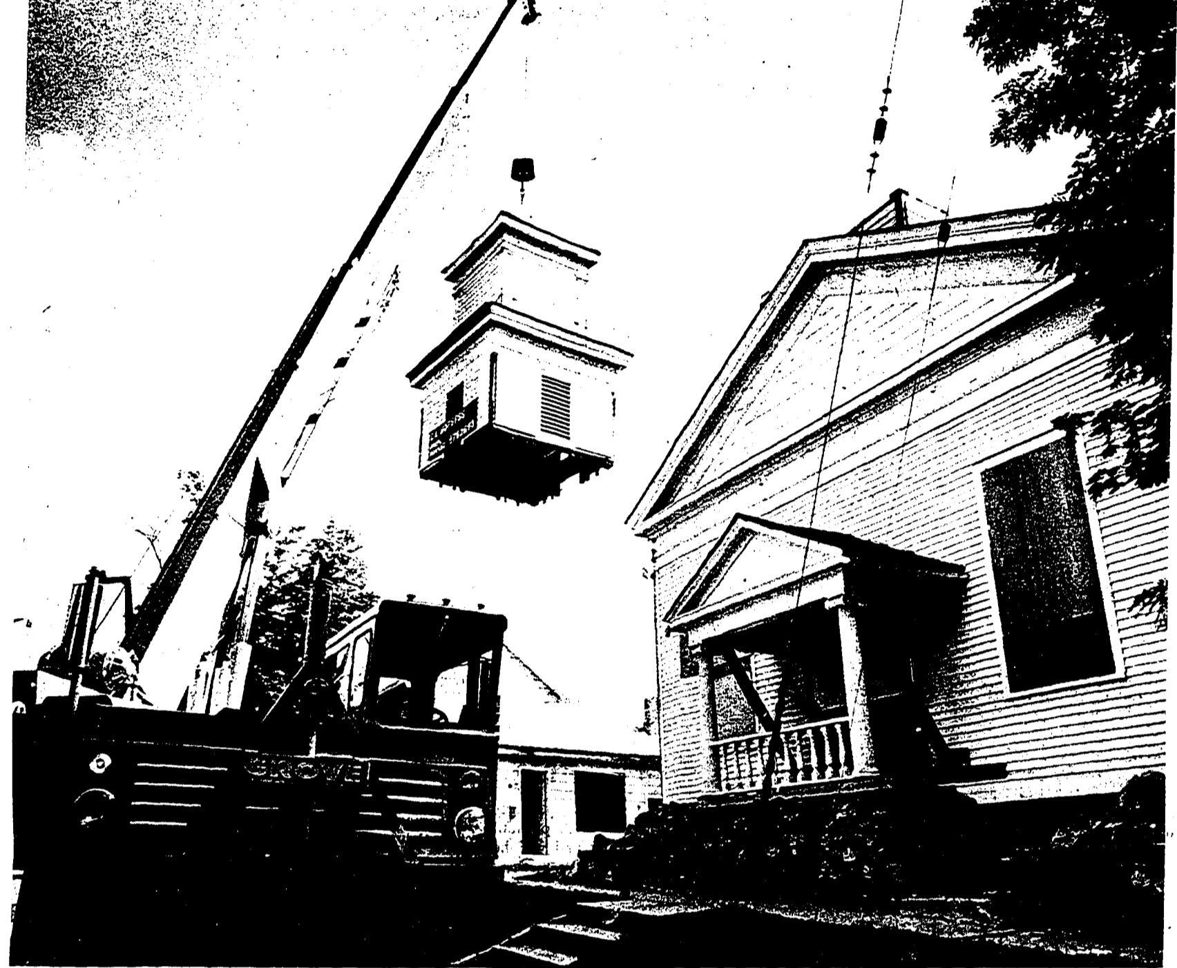
MOVE NEARS—Removal of the cupola Tuesday morning from the old library building, most recently used as the township hall, signalled the upcoming move of the historic, 125-year-old building to a new location on the west side of Griswold Street. The building is to be refurbished and turned into a community museum.
