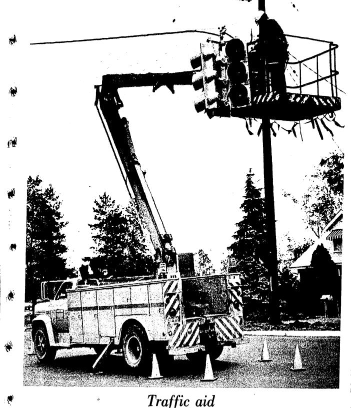
Workmen with the Oakland County Road Commission were busy installing a traffic signal at the Pontiac Trail-South Commerce Road intersection last week. The traffic signal is part of an overall intersection improvement program financed by Walled Lake and
