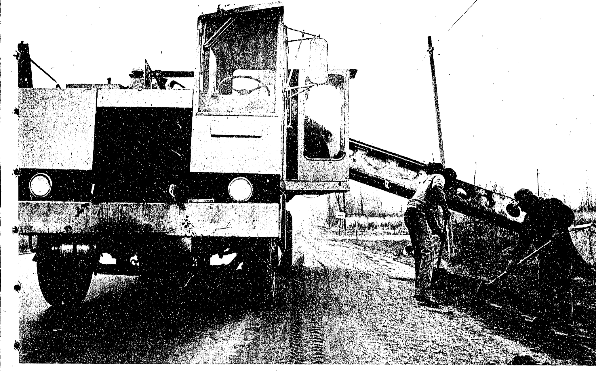
Work is proceeding on the paving of Beck Road between 10 Mile and Grand River as part of Novi's road improvement program
