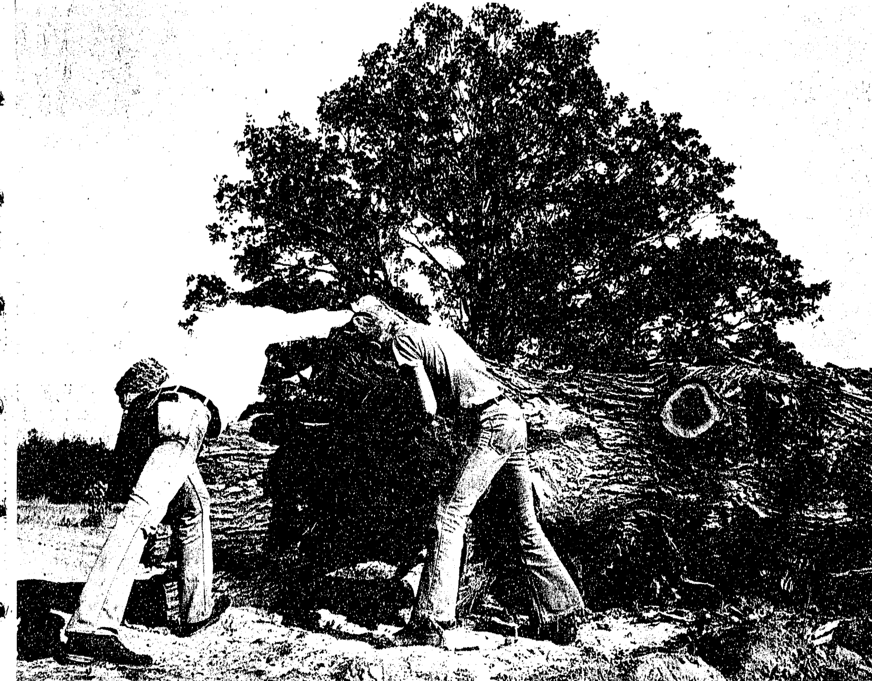
Construction workers remove a white oak stump from the Lake Pine Subdivision in Commerce Township
