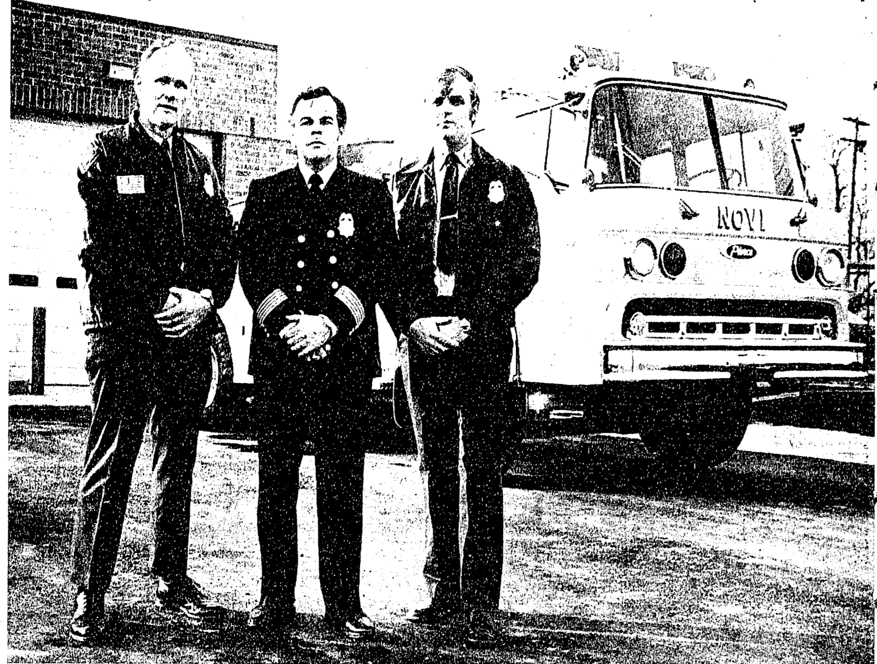
Fire hall dedicated
