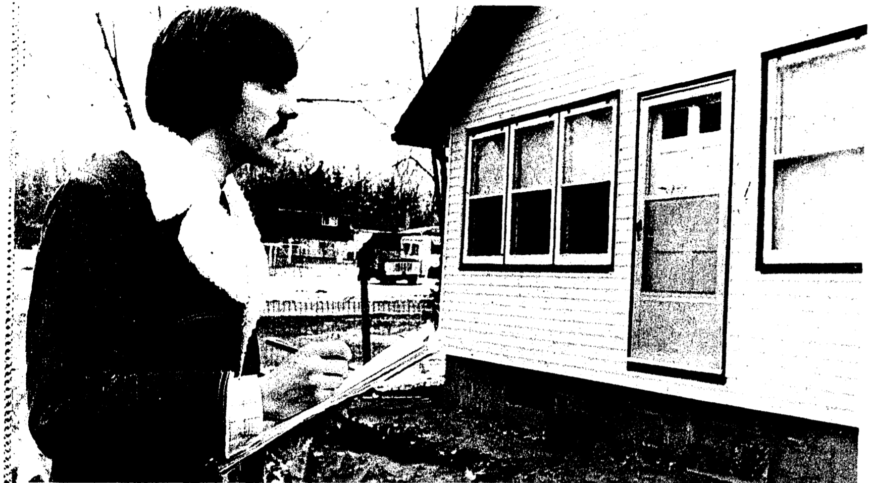
Housing Rehabilitation Coordinator John Hazelroth inspects a siding installation project (Staff photo by Jane Hale)
