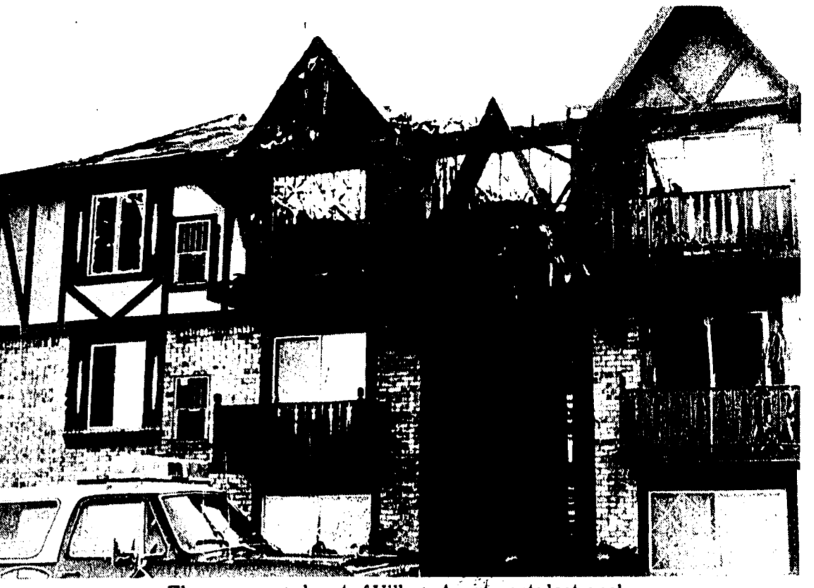
Flames ravaged part of Village Apartments last week
