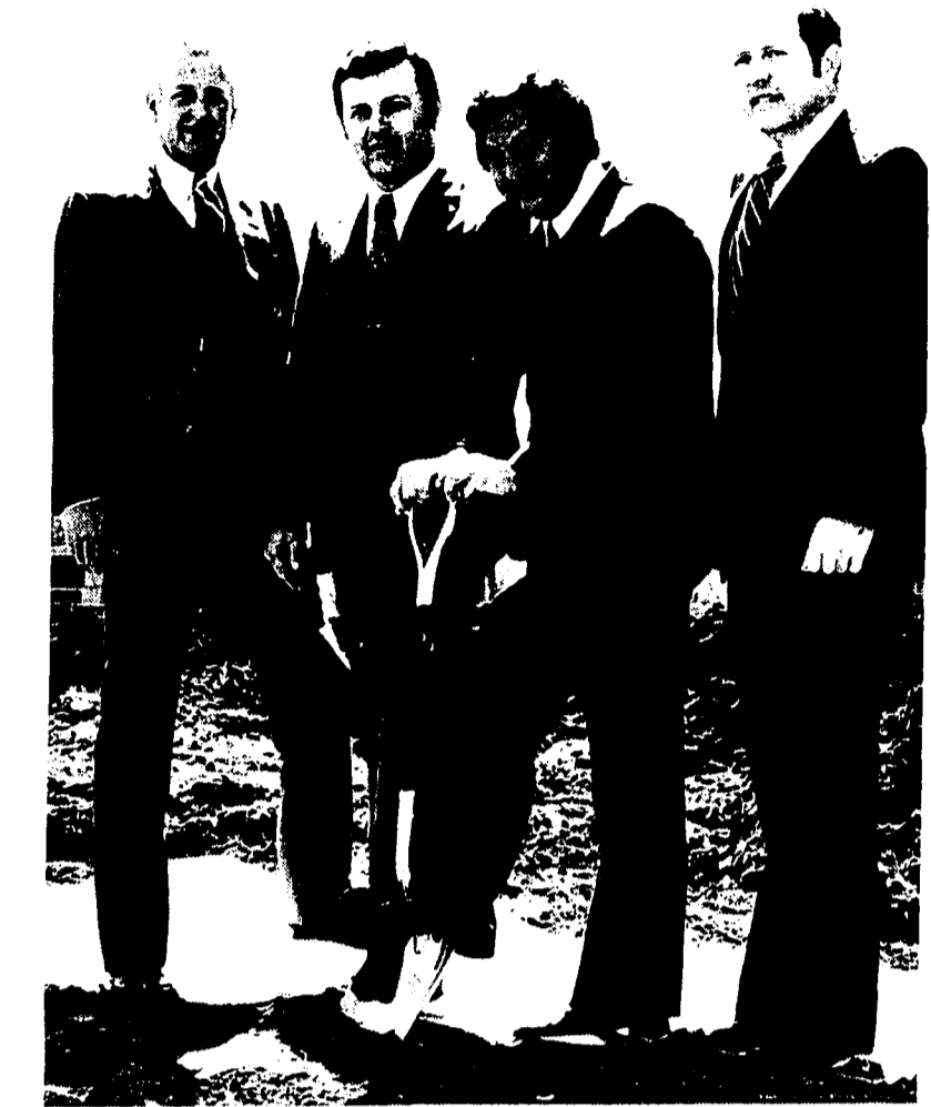
MARTY FELDMAN (second from right) breaks ground for Marty Feldman Chevrolet, Inc., on Grand River Avenue near Novi Road in Novi. The new dealership is scheduled to open in autumn this year. It will be the first completely new Chevrolet dealership in the automaker's zone since 1971.
