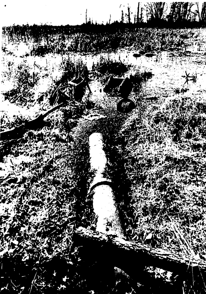
HIGH TIDE - The culvert (left) that runs off Springpark into Mud Lake is quickly immersed in the high waters. For Springpark residents, the problem continues.
