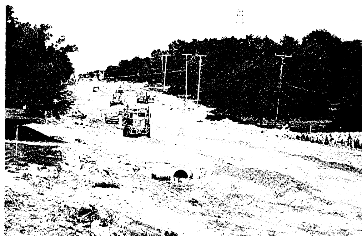
10 MILE ROAD between Telegraph and Northwestern as it looked in preparation for five new lanes of pavement.
