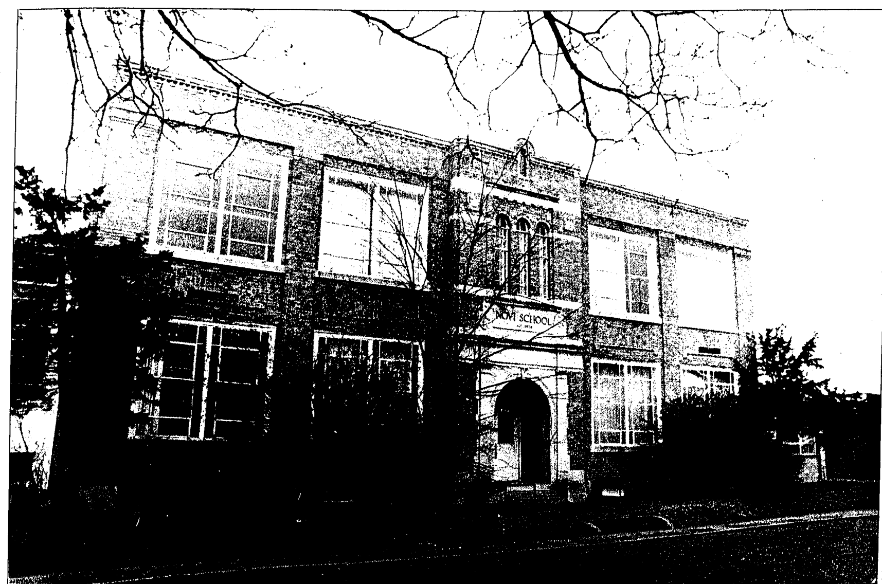
Novi Elementary School
