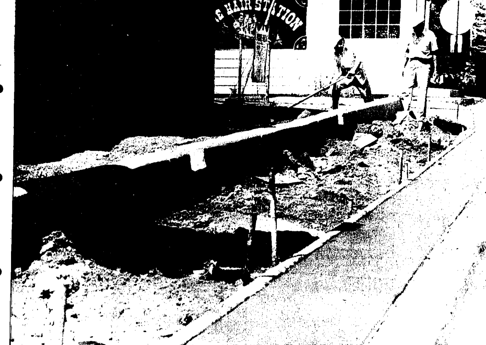
Downtown Wixom is getting a facelift as workers begin installation of new sidewalks
