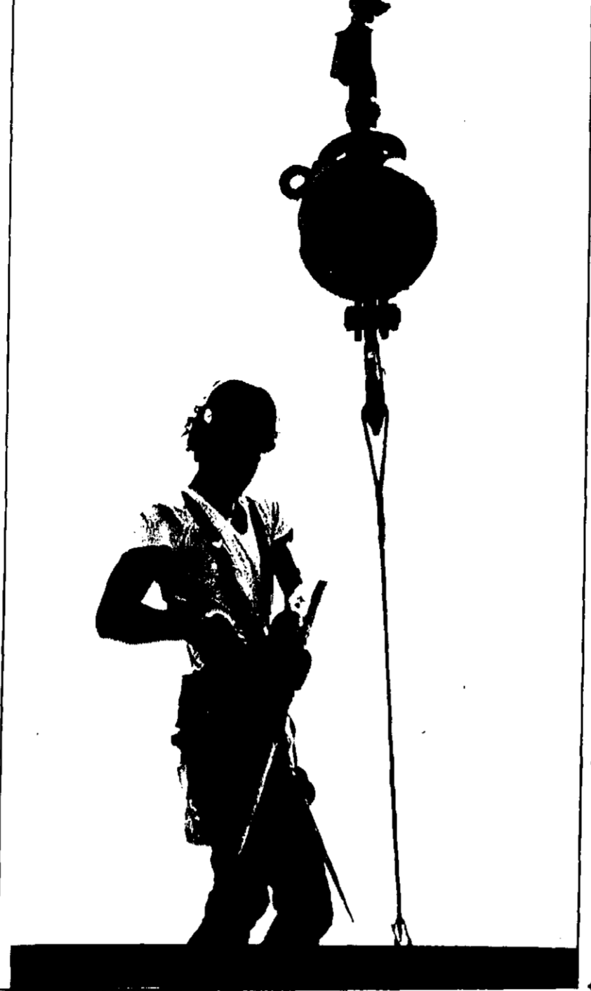
Ken Gonzalez is helping to construct the steel for the Novi Hilton under construction at Eight Mile and Haggerty Road
