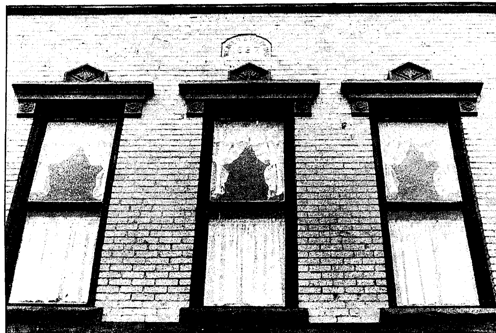
Milford blends the old (right) with the new. Builder Paul Fremling (below) stands in the new Village Center Mall, a 140,000-square-foot retail area created from two old stores.
