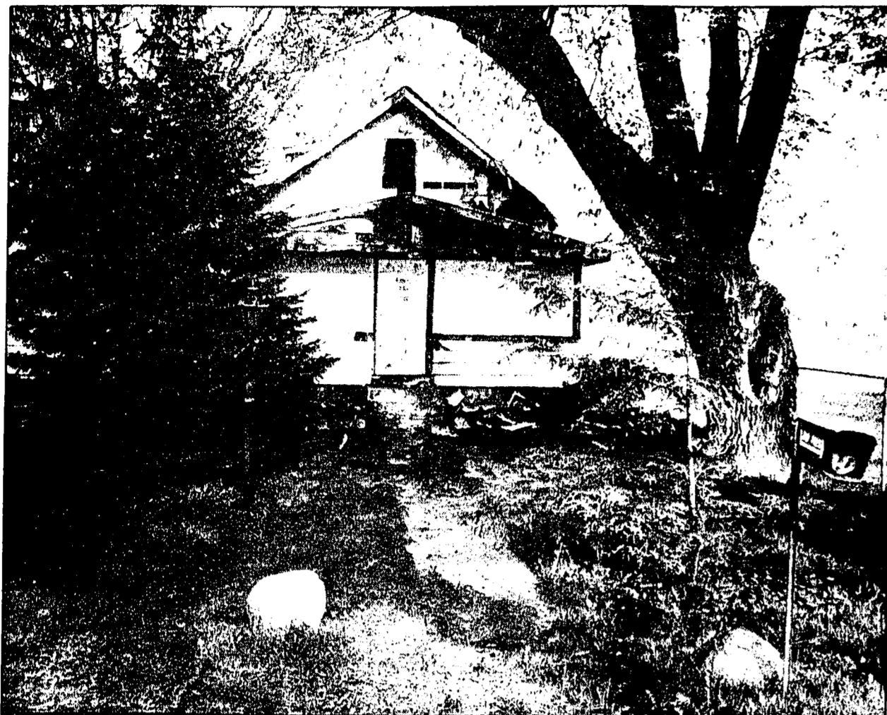
A fire caused $25,000 worth of damage to this Austin Drive home Sunday night
