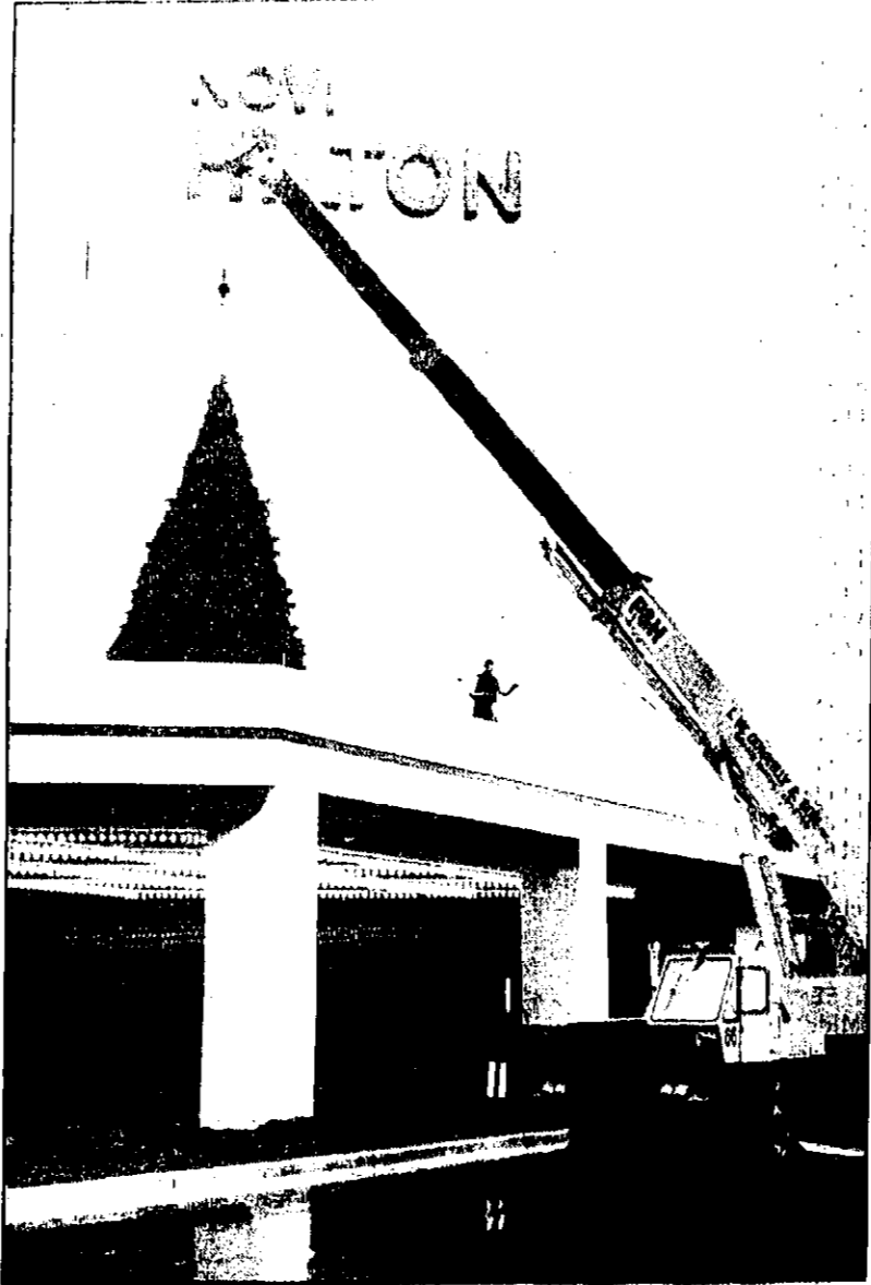
The metal-framed tree is hoisted into position on the roof. Novi News/CHRIS BOYD
