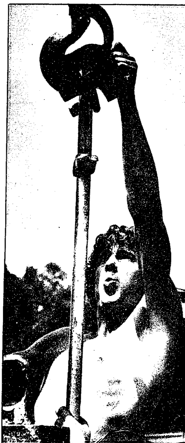
(Clockwise from upper left next to copy) John Anderson of Northville puts the first pizza of the day in the oven at the Pizza Cutter; Joe Maher, of Maher Drilling, finishes installing a 100-foot water well at Thirteen Mile Road near Decker Road; and Dennis Lee takes a break from the heat while straightening a truck frame at Harold's Frame Shop
