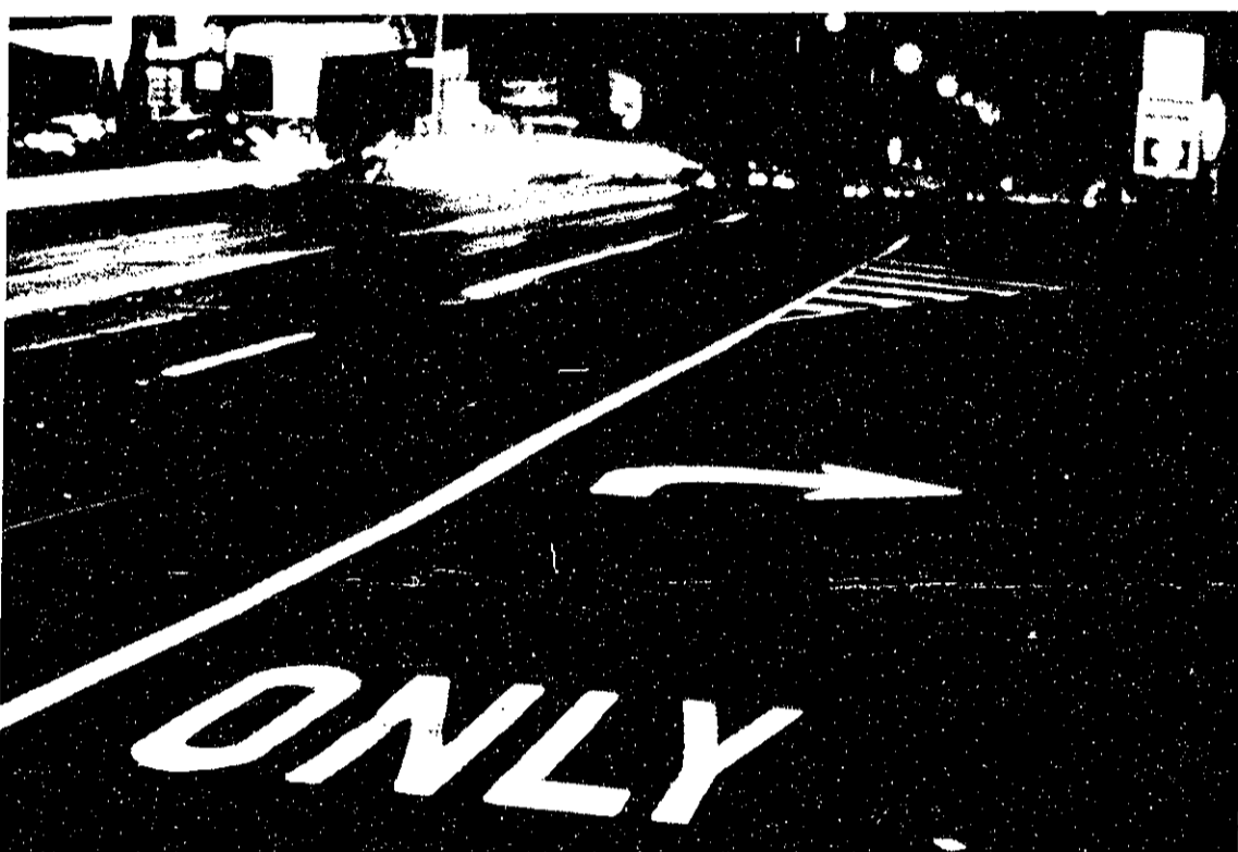
REFLECTORS GLOW — Extra safety to motorists is provided by use of reflectorized materials in signs and pavement markings.
