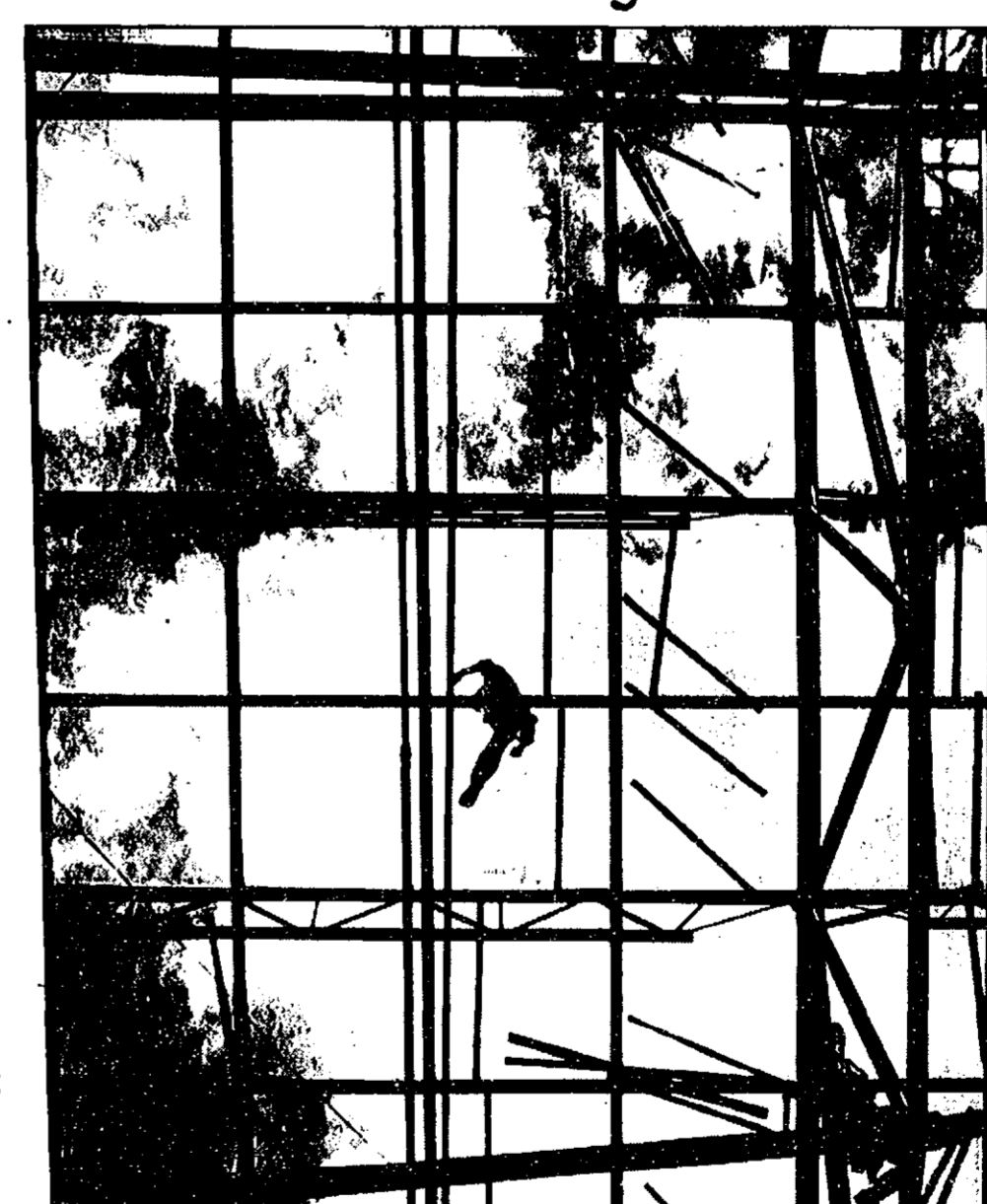
Construction workers at the new Novi Civic Center (above) worked on the building throughout the year. Late in December, city workers set up shop in the new facility.
