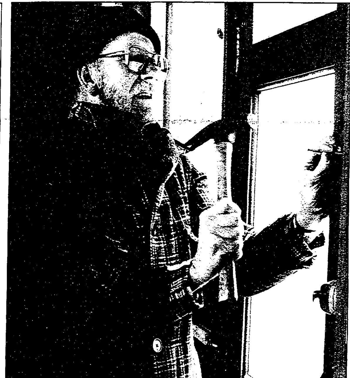
Society Member Tom Needham nails shut a door during a Town Hall work bee last Saturday
