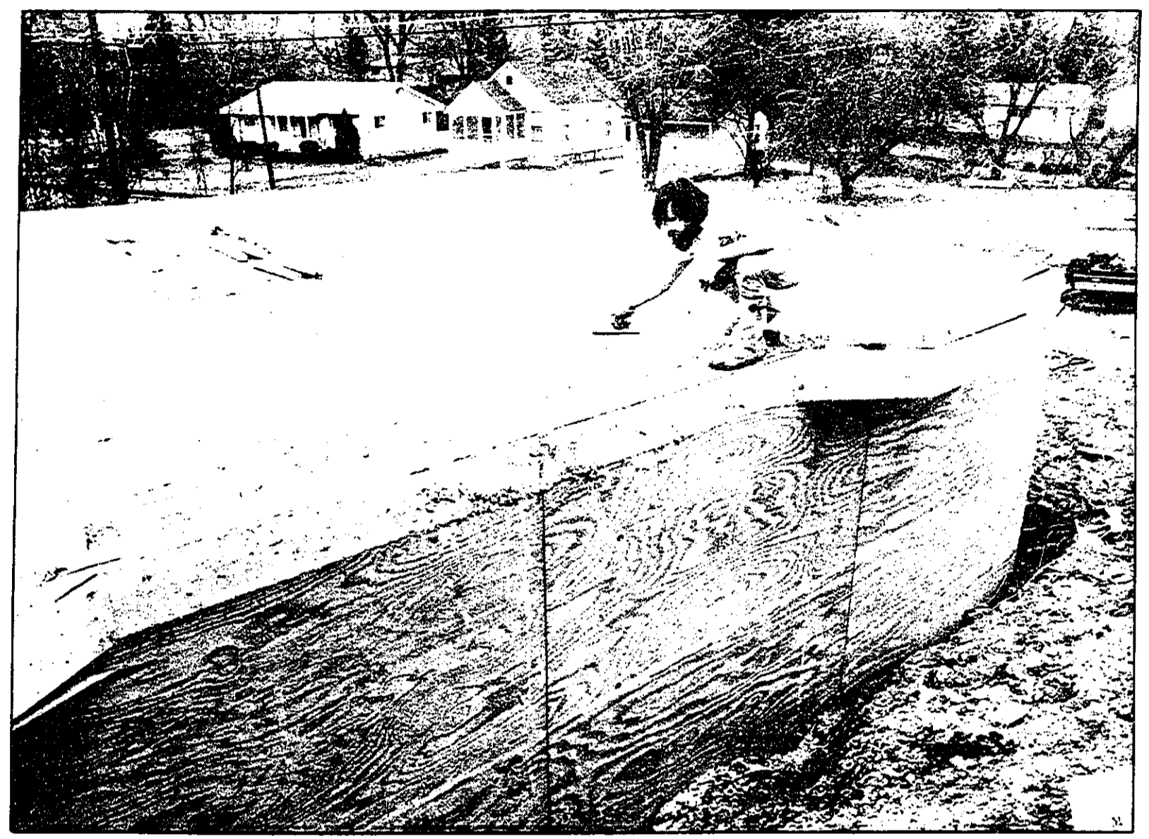
Bill Gourlay smooths out the cement floor built atop a wooden foundation in an Integral Works home. Photo by CHRIS BLOYD
