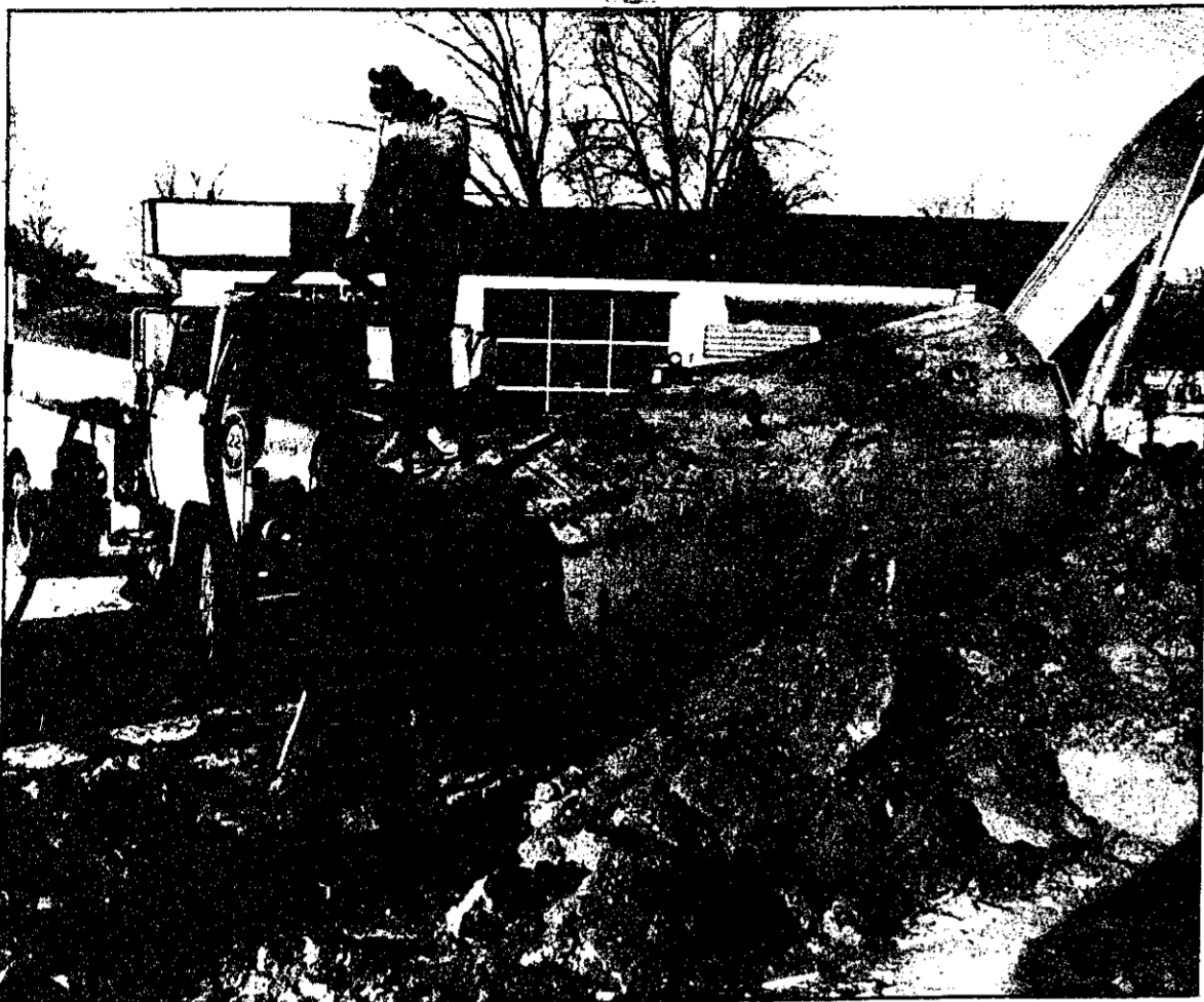
Workers remove empty tanks from the former gas station on Novi Road at Thirteen Mile
