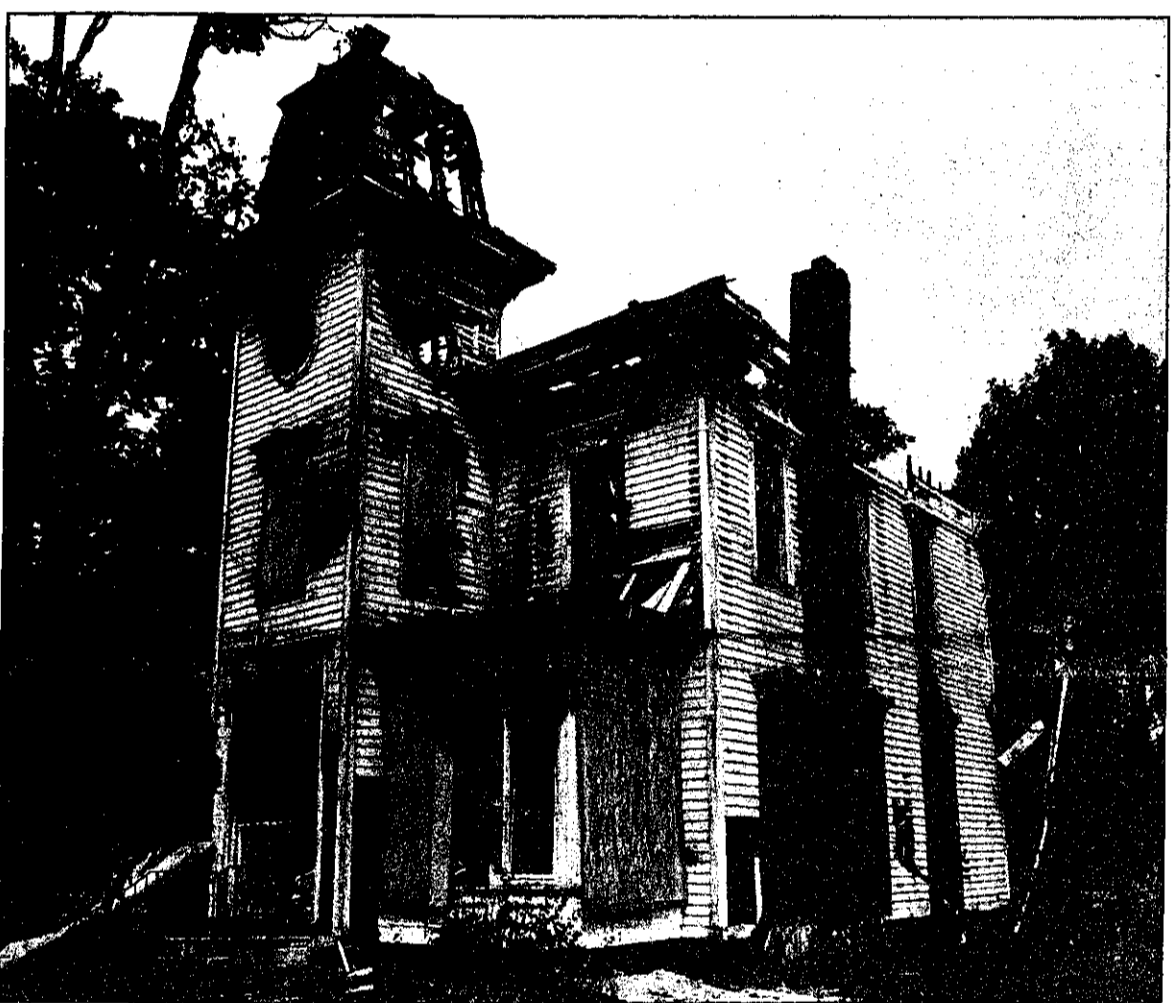
Flames destroyed Novi's historic Yerkes House early last Thursday morning
