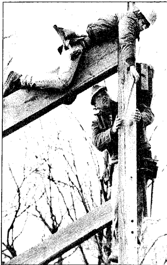
Construction workers install a beam
