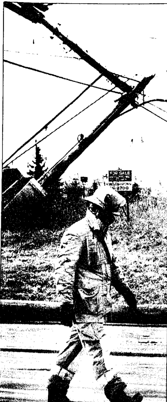
A Farmington Hills fireman walks past the utility pole that was struck by a truck during an accident at the Nine Mile/Haggerty Road intersection last Monday.
