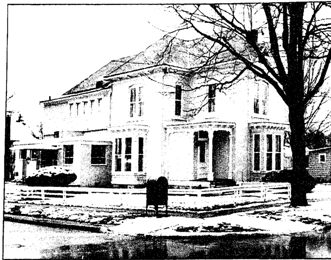
This Northville house was converted from a doctor's office to a bed-and-breakfast inn.
