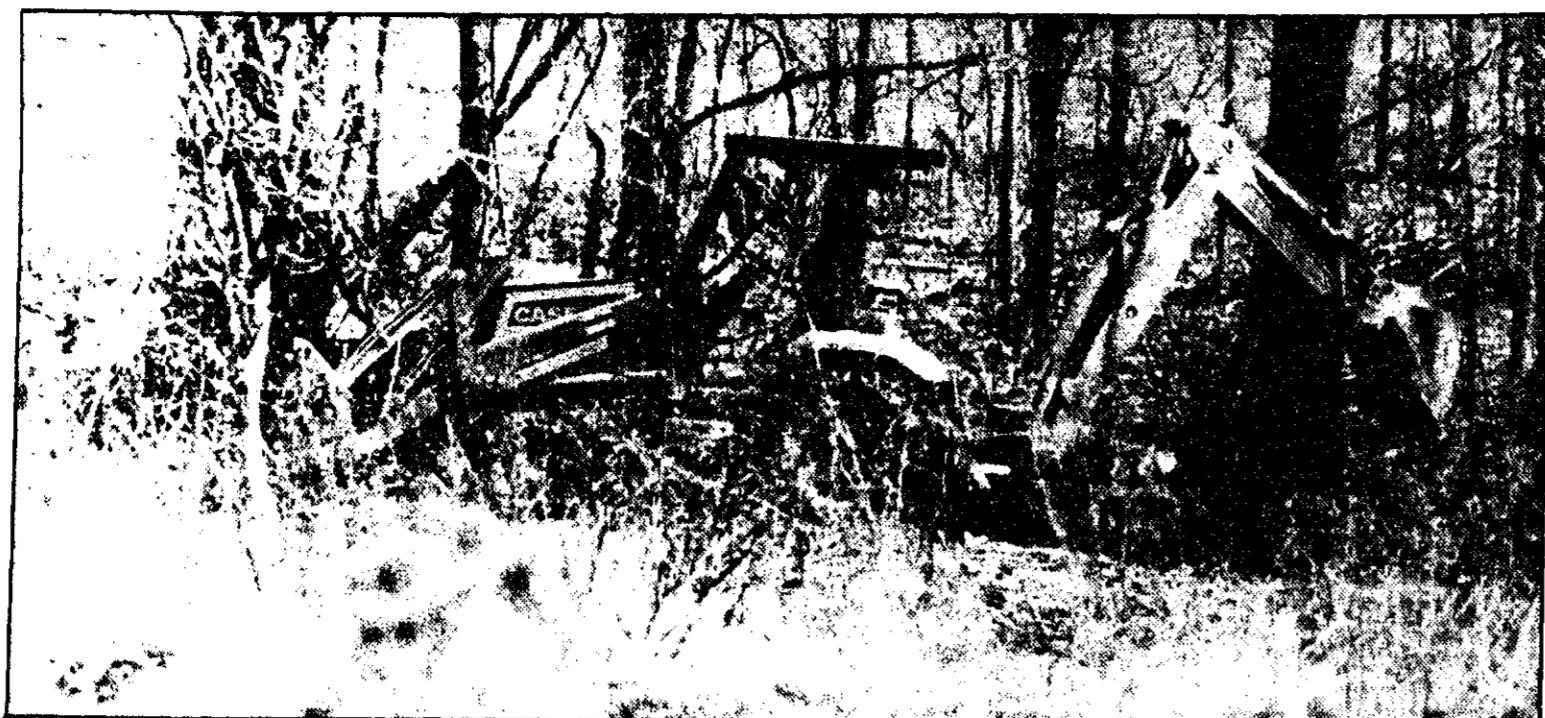
A backhoe digs a drainage trench April 27
