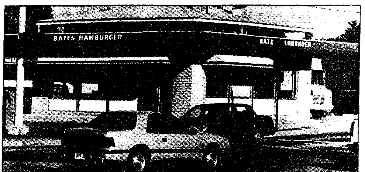
Existing buildings, such as Bates Hamburger, pose problems for city planners in devising the town center scheme. The challenge is to design the town center so that the older buildings fit.
