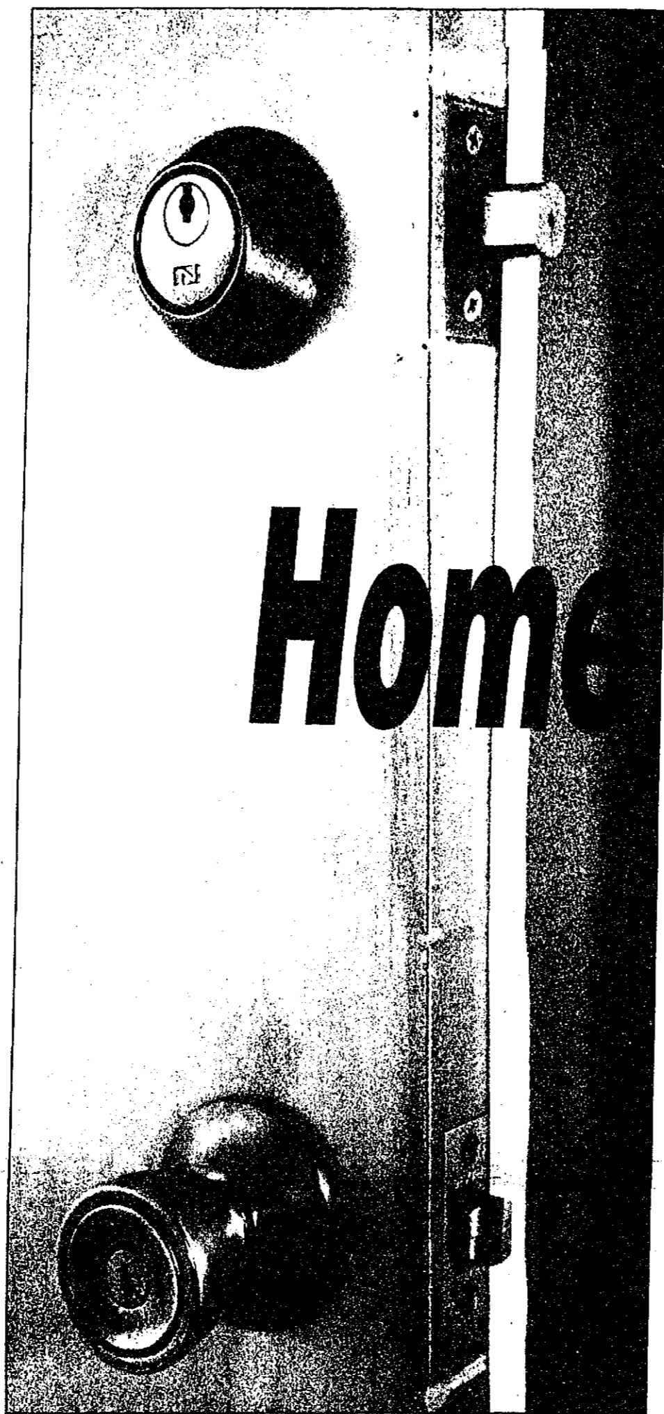
The top lock is a good example of a strong deadbolt.
