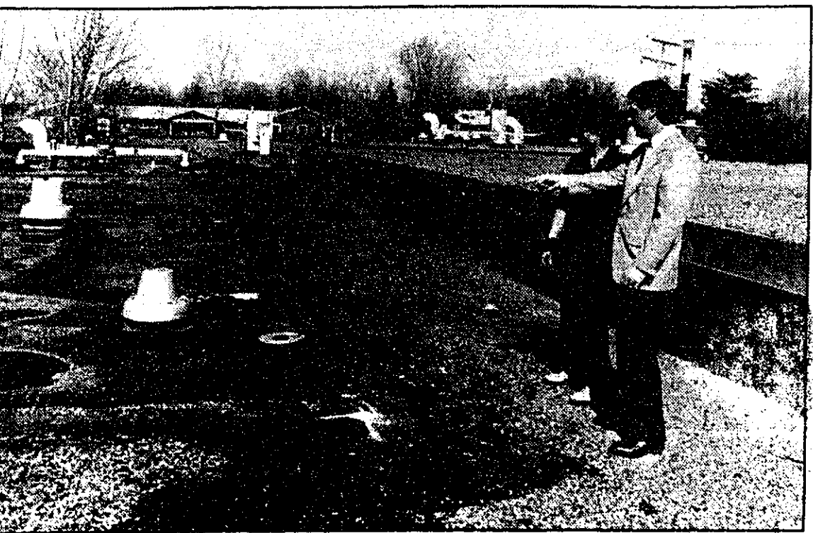
Above, Sandy Spiro and maintenance man Jeff Anderson inspect the roof that will be replaced. At right, Jack Farley of Clark Painting prepares for a painting project at the center.
