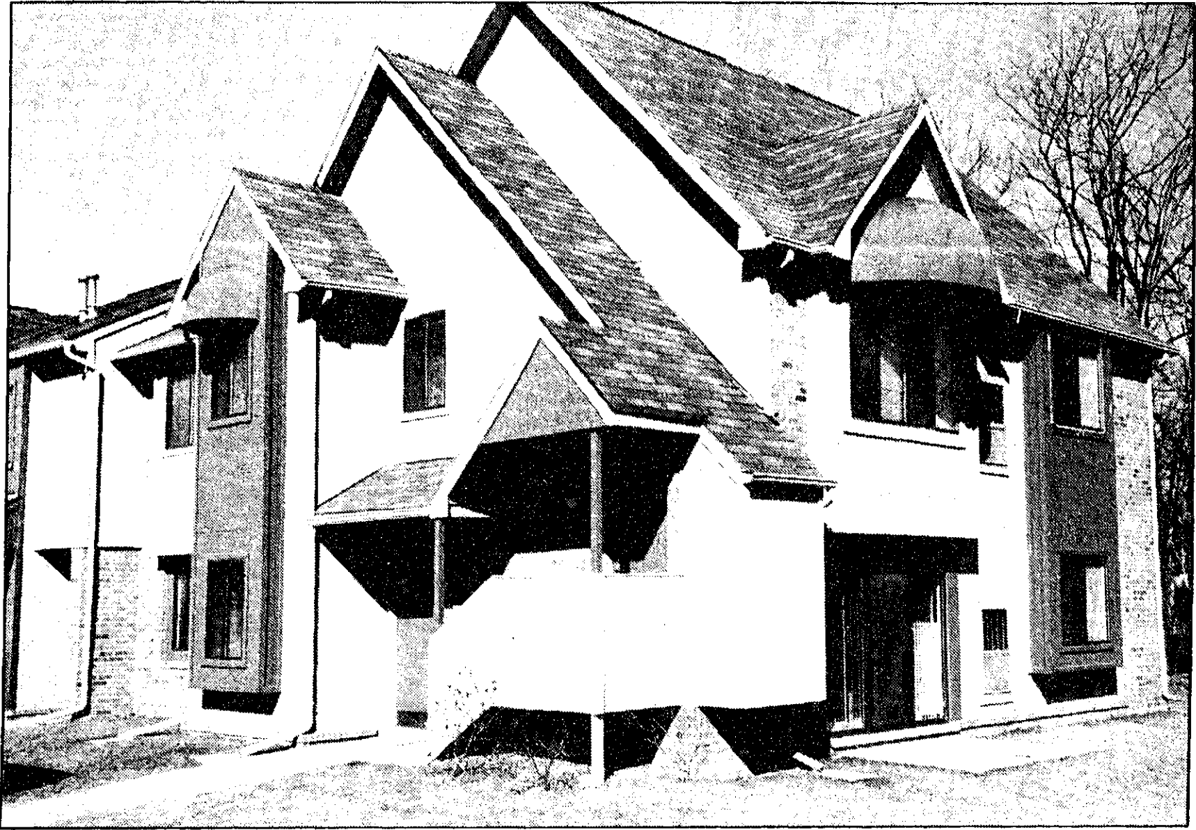
Awnings at Polo Club Apartments in Farmington Hills coordinate the paint scheme and save on cooling costs
