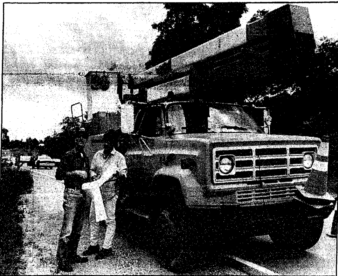
A Detroit Edison crew checks out the hot, downed line
