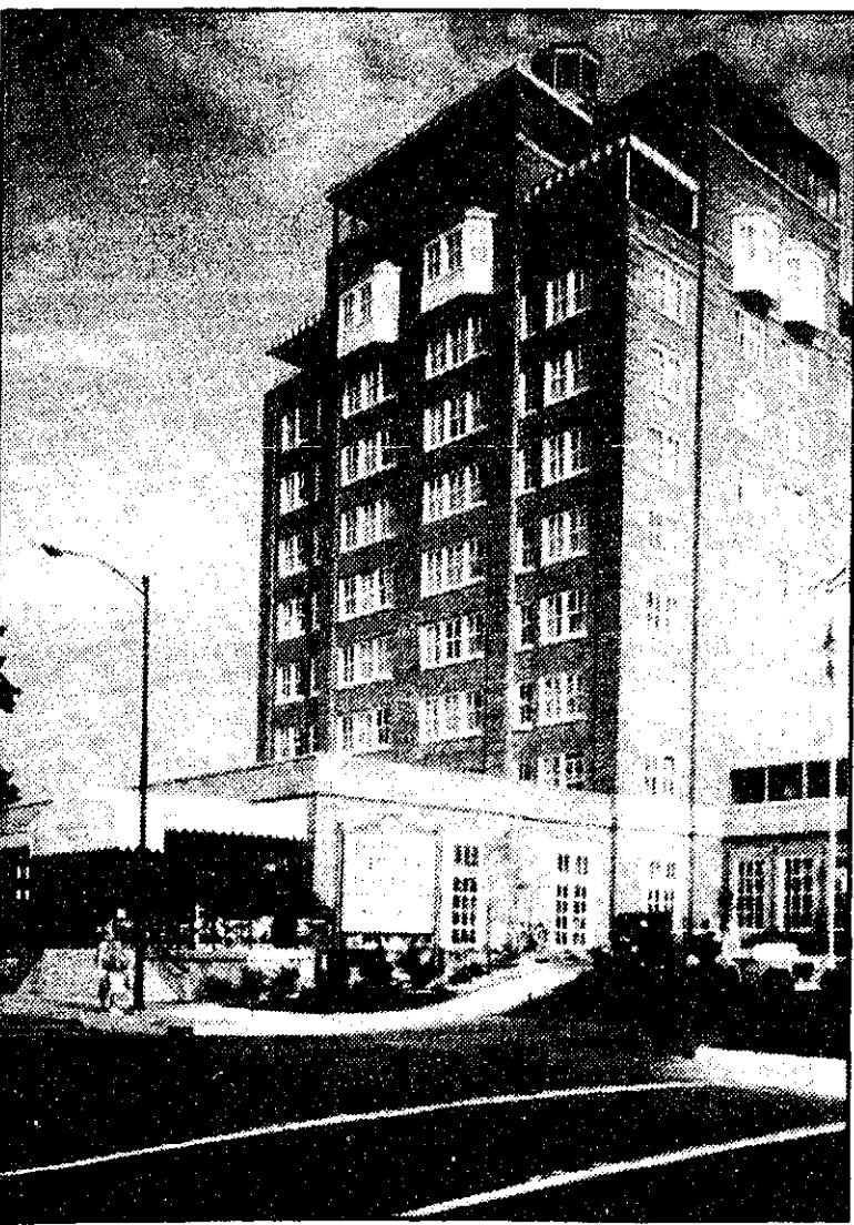
Traverse City's Park Place Hotel has been completely renovated
