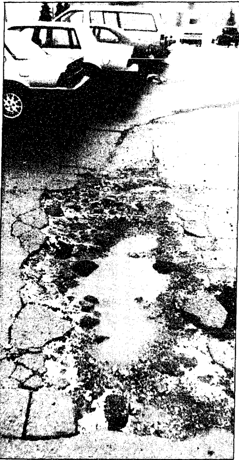
"The" pothole in the library parking lot.
