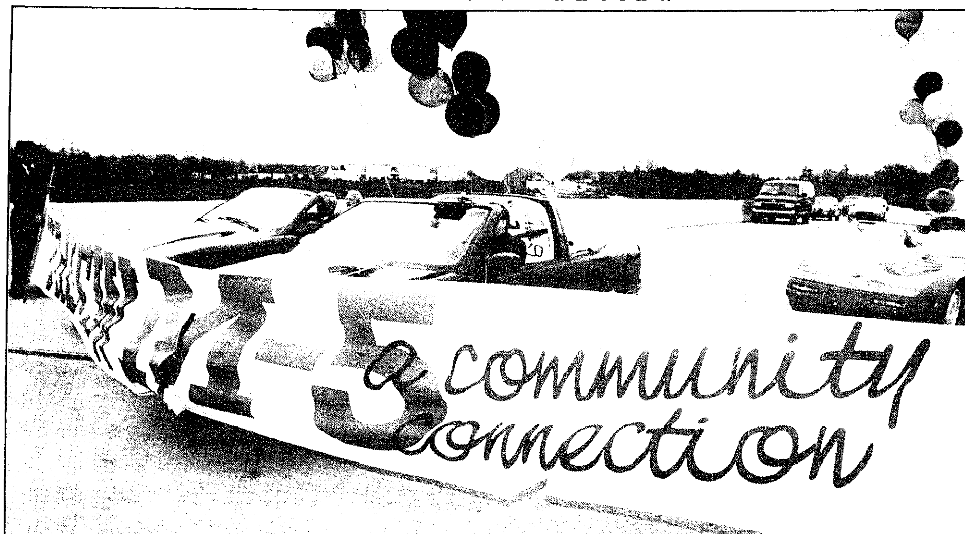
The $35 million Haggerty Connector interchange, linking I-96, I-275 and southbound M-5 with Twelve Mile, was opened with much fanfare in October.
