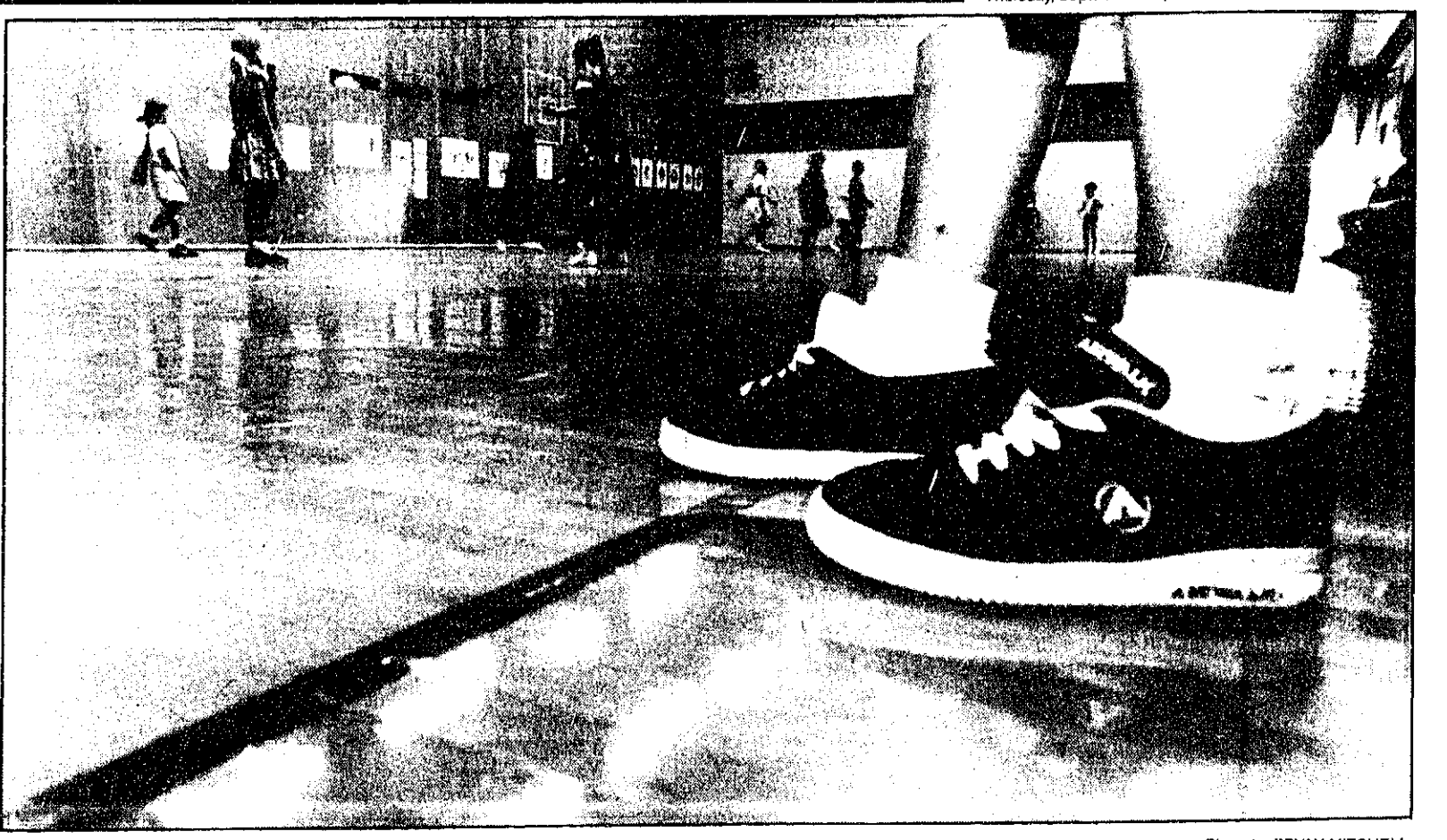
A leaky roof at Novi Meadows is causing the gym floor to bubble. Photo by BRYAN MITCHELL.
