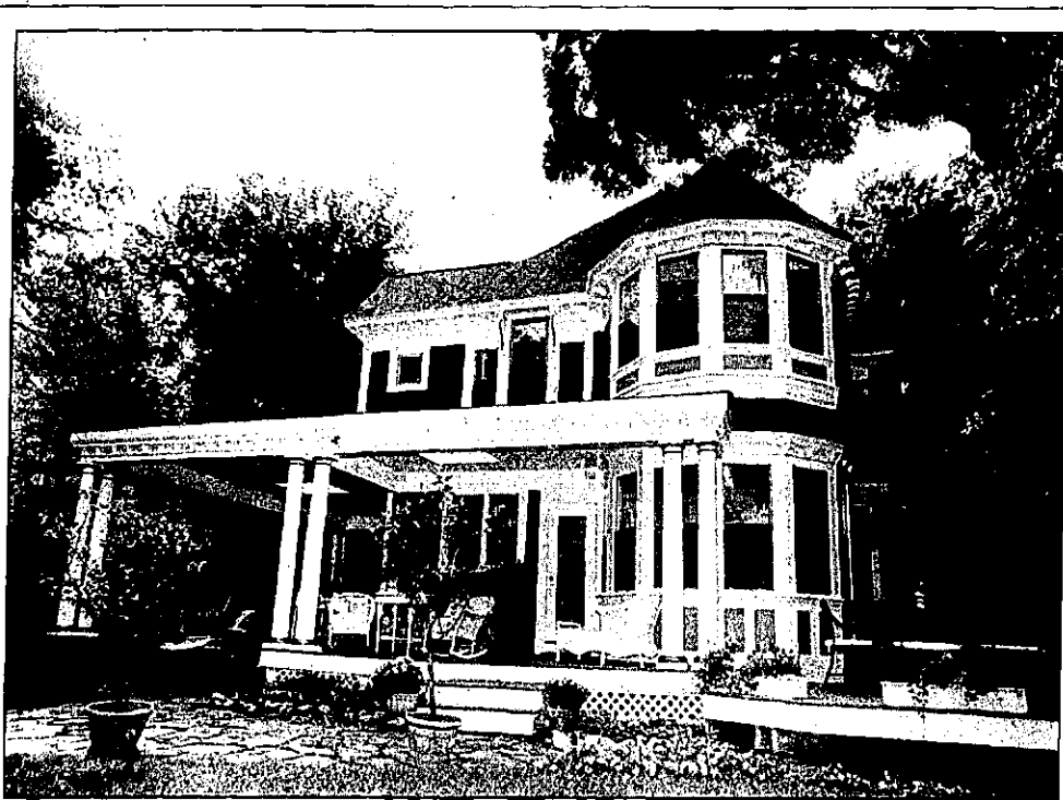
Photo by BRYAN MITCHELL Additions to the back of the house included a two-story turret, windows, a one car porte-cochere, and wrap-around veranda with a screen porch area.
