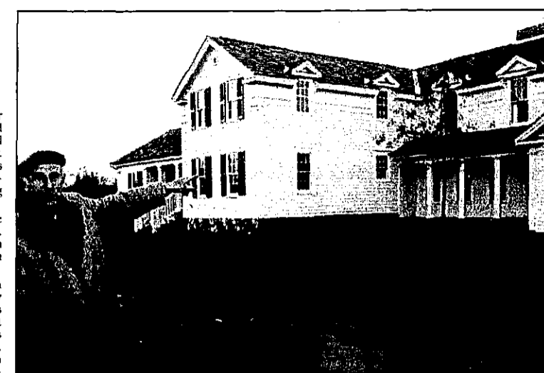
Bill Garfield stands outside the almost-remodeled and finished Sally Thornton House.
