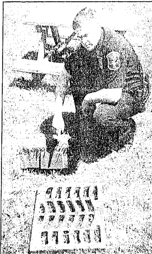
Northville Fire Sgt. Michael O'Brian points out the sewer into which a Northville toddler fell Monday. Quick action by the child's mother averted a tragedy. Officials speculate teens may have removed the manhole cover as a prank.
