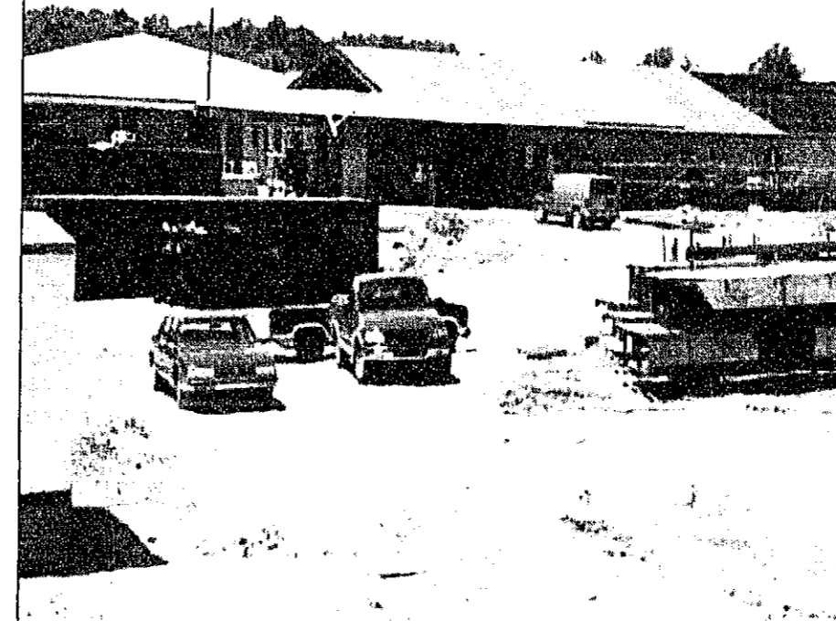
Construction of the new Middle School, part of the honored land deal, is moving ahead. Photo by JOHN HEIDER
